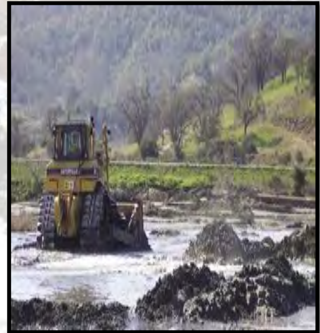
e.g., dredge and fill
